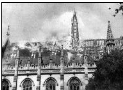
Wilson Hall burning down, 25 January 1952 (UMA photo no. 613). Although the building and contents were insured for £100,000, there was considerable loss of irreplaceable artworks, furniture and papers.
